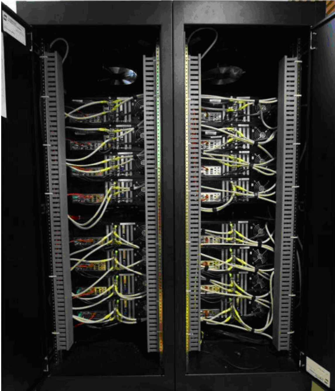
Figure 2.8: Back view of the PC-Cluster showing the wiring interconnecting the 16-Nodes
