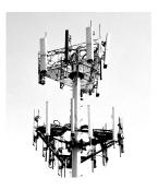
Space diversity is also used by many point-to-point microwave links by placing two antennas separated vertically on the same tower.
