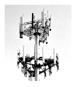
Space diversity is also used by many point-to-point microwave links by placing two antennas separated vertically on the same tower.
